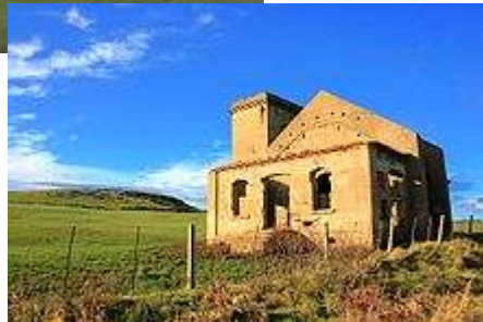
Ruins of Fan House, Huntcliff Ironstone Mine. The mine entrance went under the Cleveland Railway which still runs alongside to carry potash trains from the Boulby Mine.
