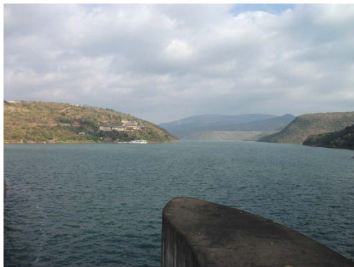
Jozini Dam (above),
